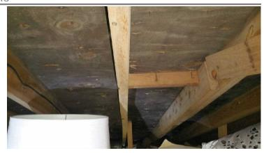
4. Overhead Attic Ventilation: Ridge vents and soffit vents - The venting in this attic is insufficient. The gable louvers are small and the soffit venting is minimal. The fan will run excessively and the dark roof sheathing is a by-product of bad venting. Consider adding more venting both low and high.
